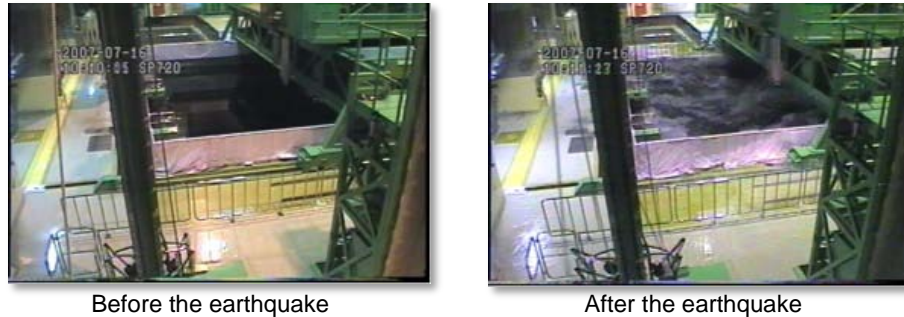
Fig. 6-1 State of the spent fuel pool of Unit 3 of the Kashiwazaki Kariwa Nuclear Power Station before and after the earthquake (Source: TEPCO)
